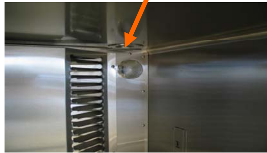
Interior view of the port
